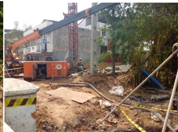
Figure 5: Bridge construction area
