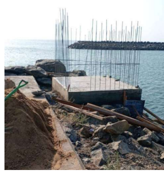
Figure 09: Ongoing Construction for new tidal and wave monitoring stations at Dondra fisheries harbor under the collaboration of South China Sea Institute of Oceanology (SCSIO), China.
