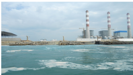
Outlet culverts of the power plant
